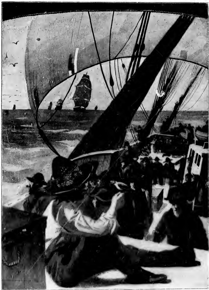
ON THE HURRICANE DECK OF THE "ACAPULCO."
